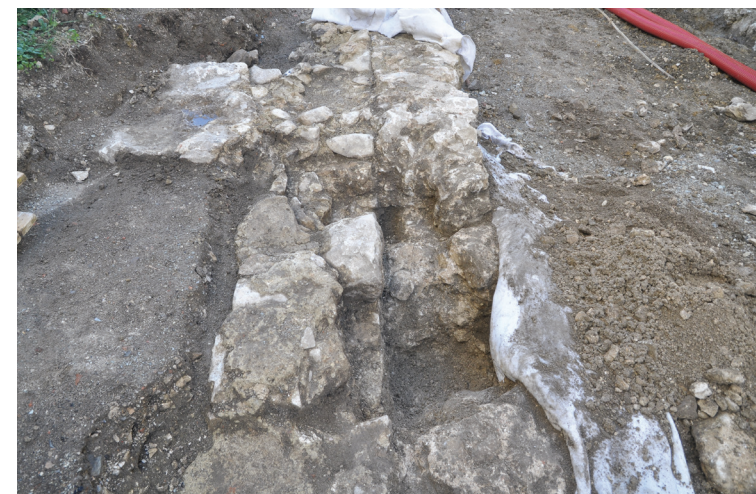
Pokopališki zid z utrditvijo / Cemetery wall and its fortification
